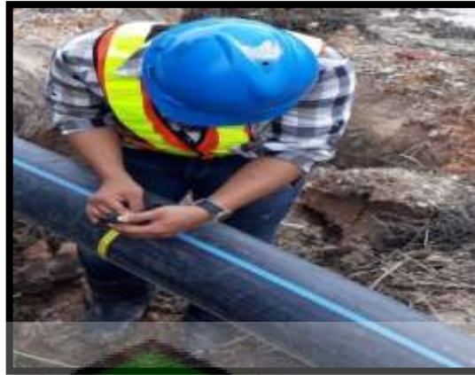
Gambar 4.5 Pengukuran diameter pipa HDPE
